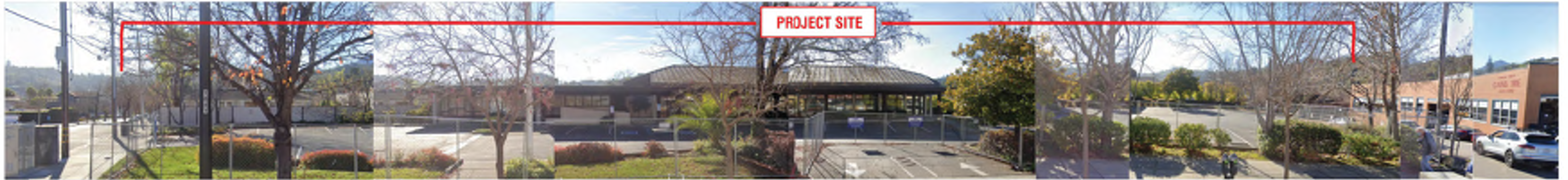
1. VIEW FROM 4TH STREET - SOUTH FACING
